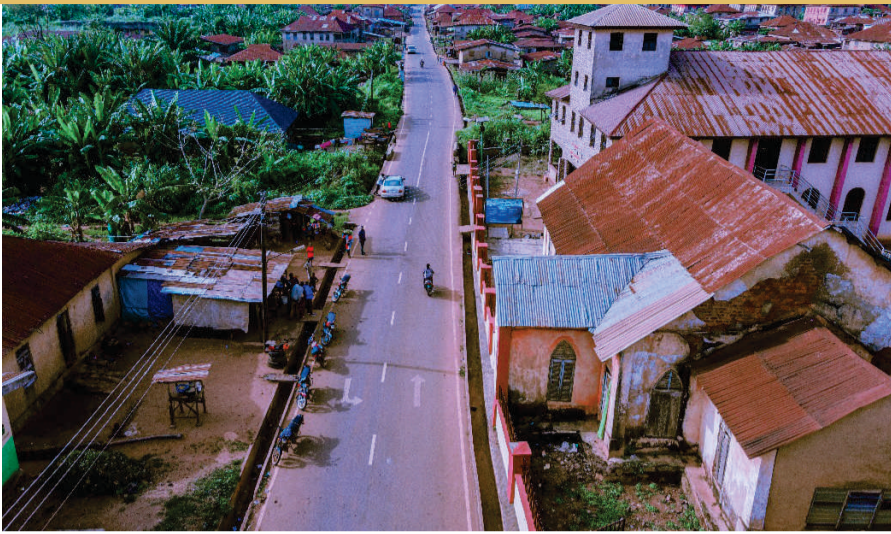
Completed Enuwa-Oniyangi-Palace road in Ile-Ife
