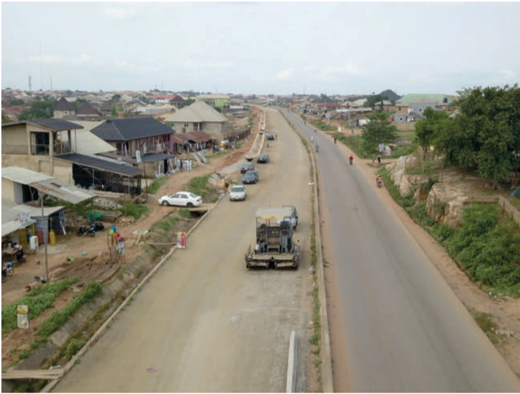
Construction of the second lane of Osogbo circular road.
