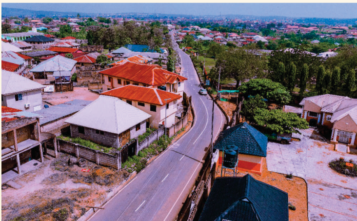
A completed road by Adeleke administration in Ikire, Irewole local government area of the State.
