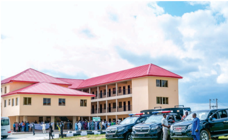
Outside view of the completed Office and lecture rooms at the Health Sciences faculty of Osun State University, Isale-Osun, Osogbo.
