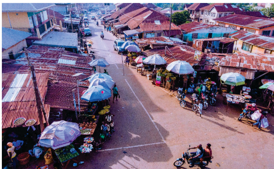
A completed road in Ilesa.
