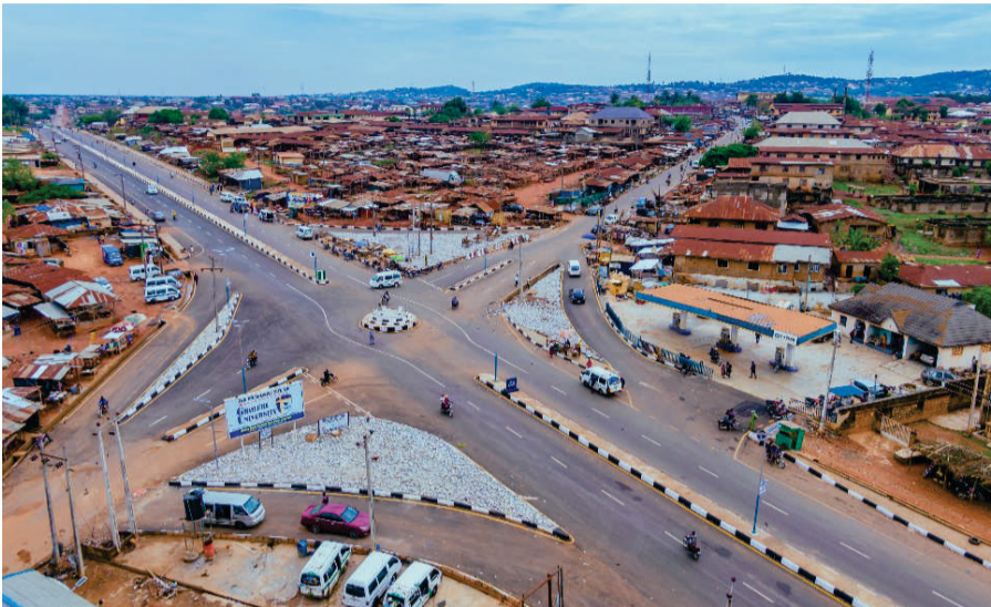
Completed section of Osogbo – Ikirun road inherited from previous administration.
