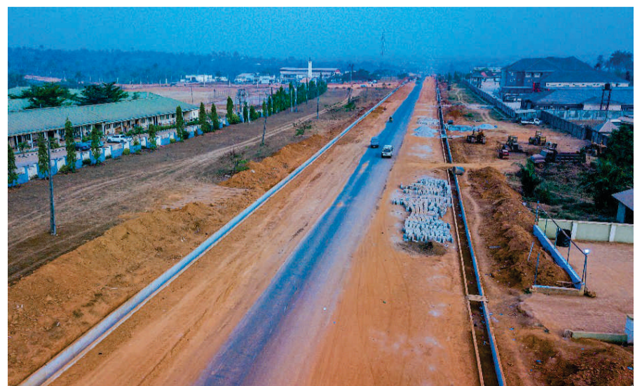
Ongoing dualisation of Akoda-Okegada road in Ede
