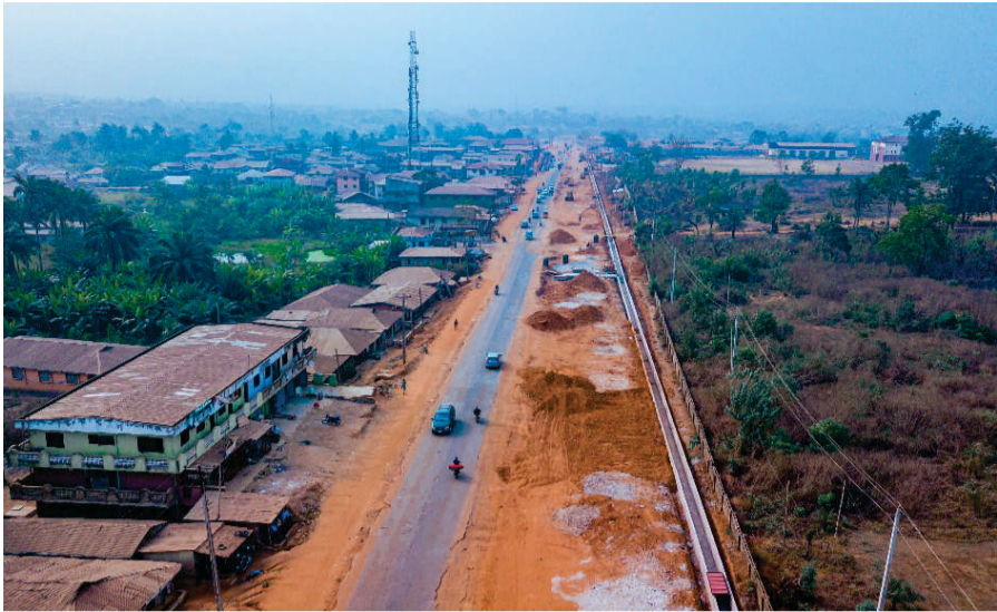
Another section of the ongoing Akoda-Okegada road.
